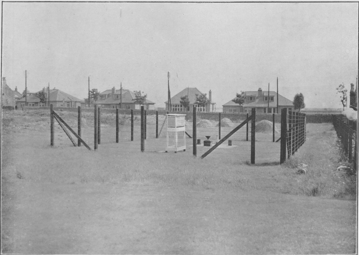
FIG. 9. NEW ENCLOSURE FOR STEVENSON SCREEN AND RAINGAUGE (seen from W.S.W.)
