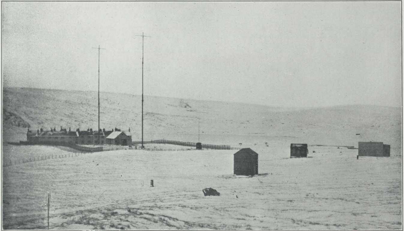
FIG. 3. GENERAL VIEW FROM SOUTH.
